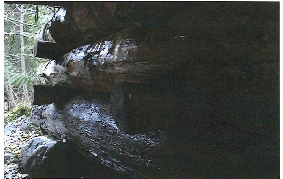
CK2304 Right Abutment
