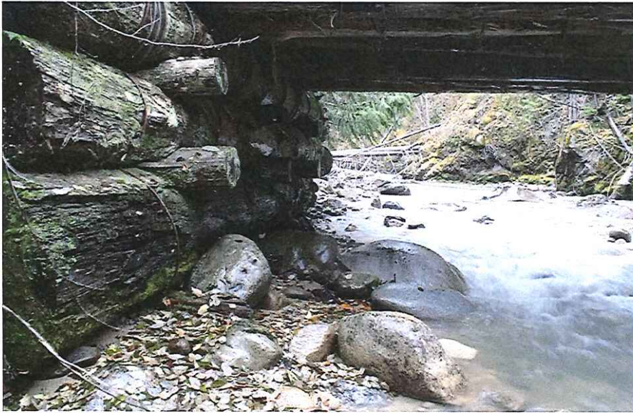
CK2304 Right Abutment 2
